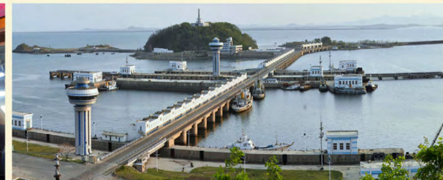
The 8km-long West Sea Barrage was built in five years.
