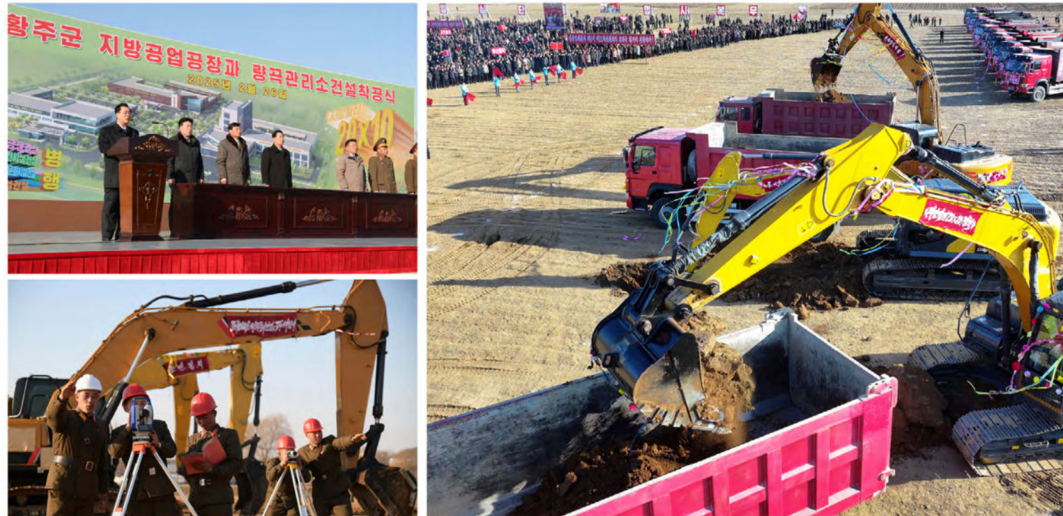
Regional-industry factories and grain storage station in Hwangju County
