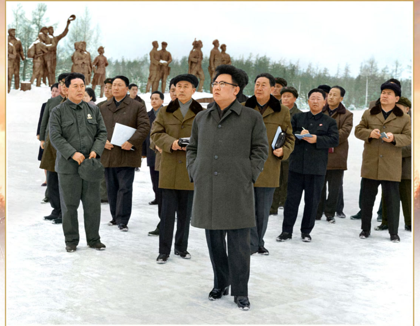
The great leader Comrade Kim Jong Il providing guidance at the construction site of the Samjiyon Grand Monument in March 1979
