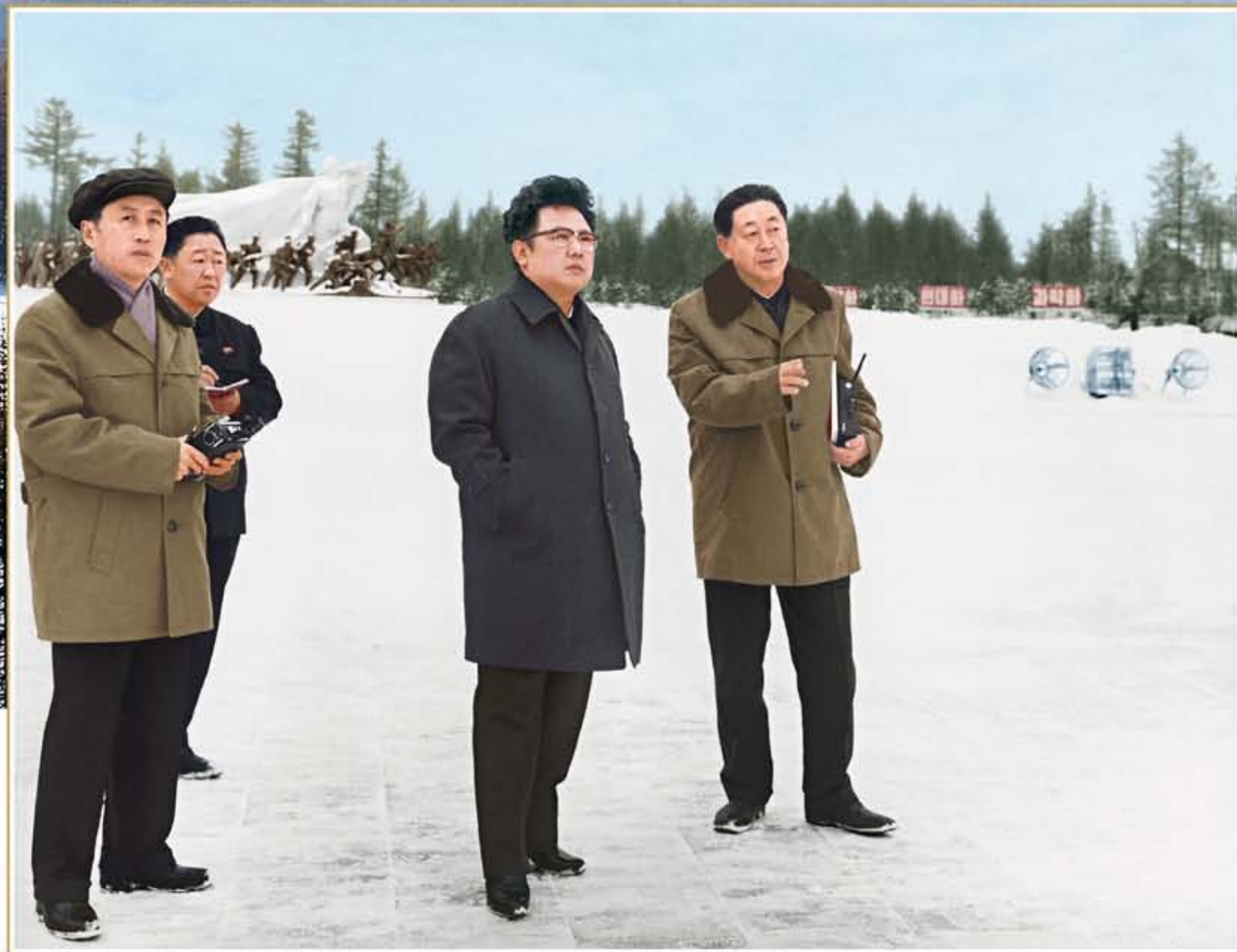
Kim Jong Il giving on-site guidance to the construction project of the Samjiyon Grand Monument in March 1979
