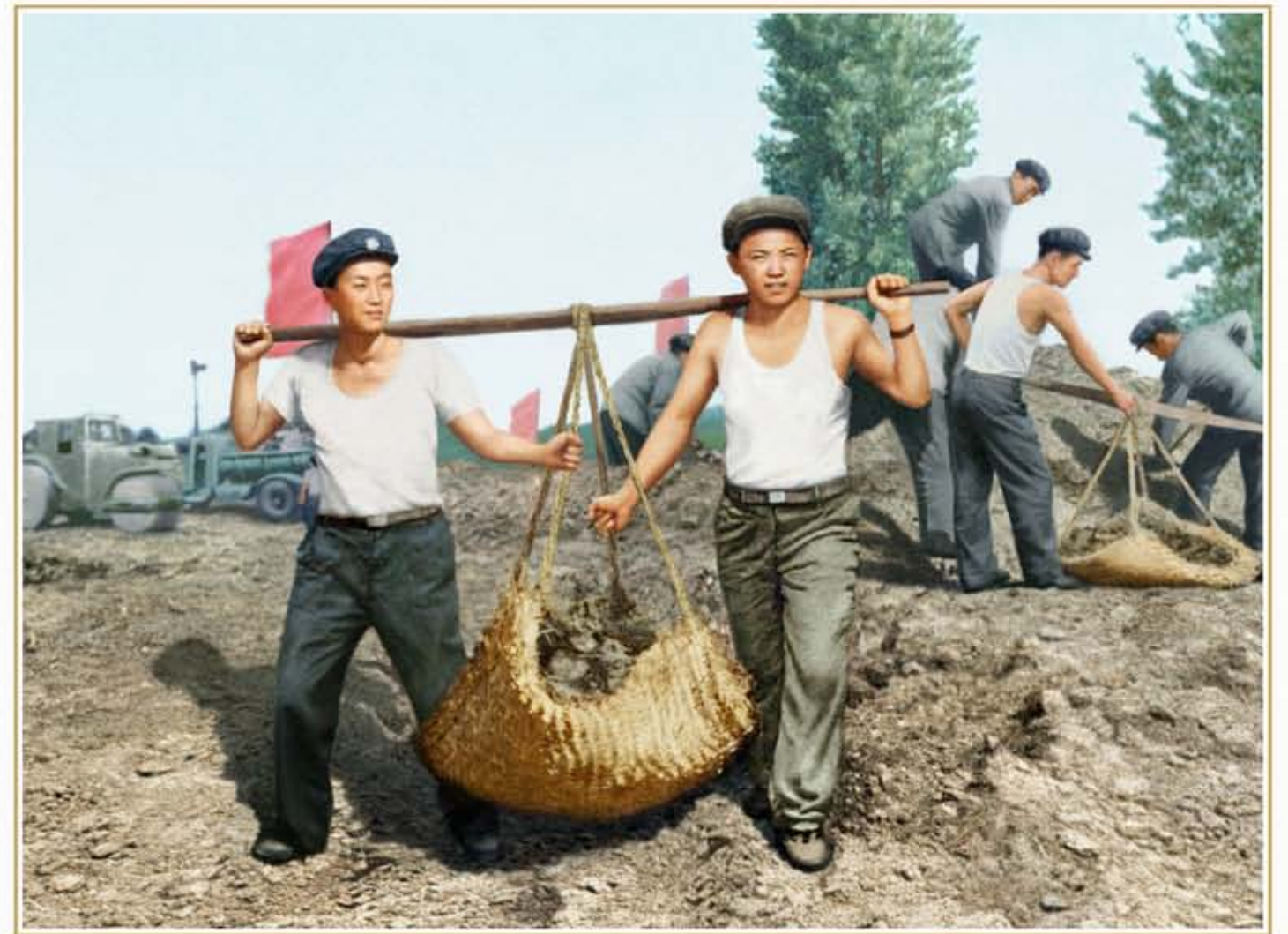
Kim Jong Il working on the project to widen the road between Wasan-dong and Ryongsong in Pyongyang in May 1961
