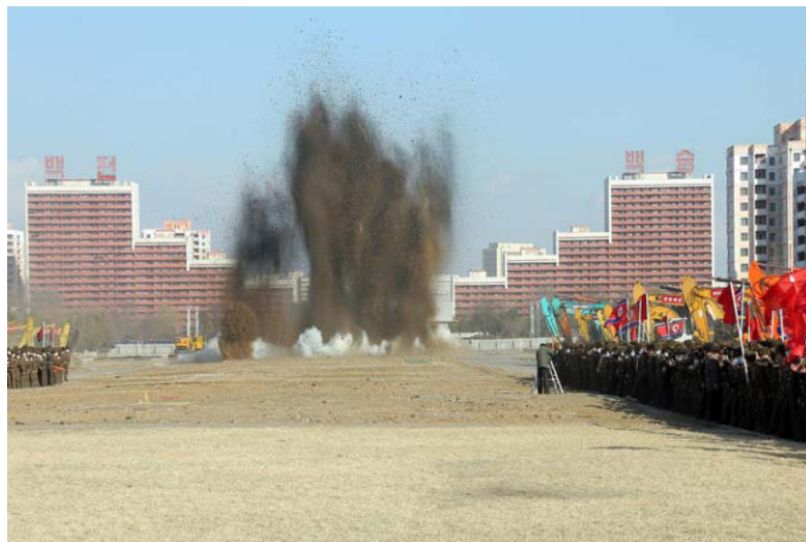
Ground-breaking ceremony of the Pyongyang General Hospital
