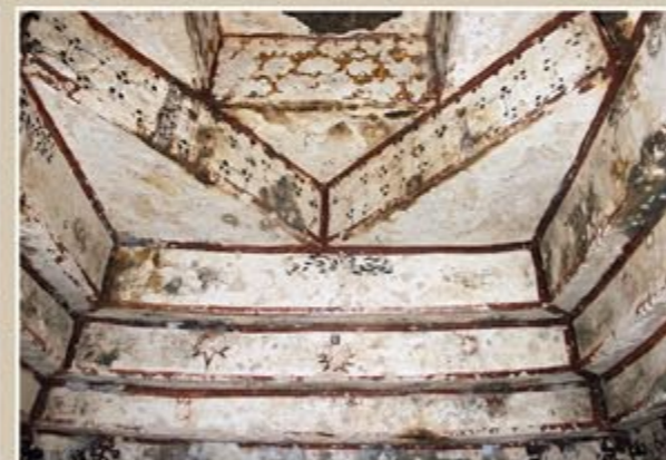
Ceiling of parallel triangular prop
