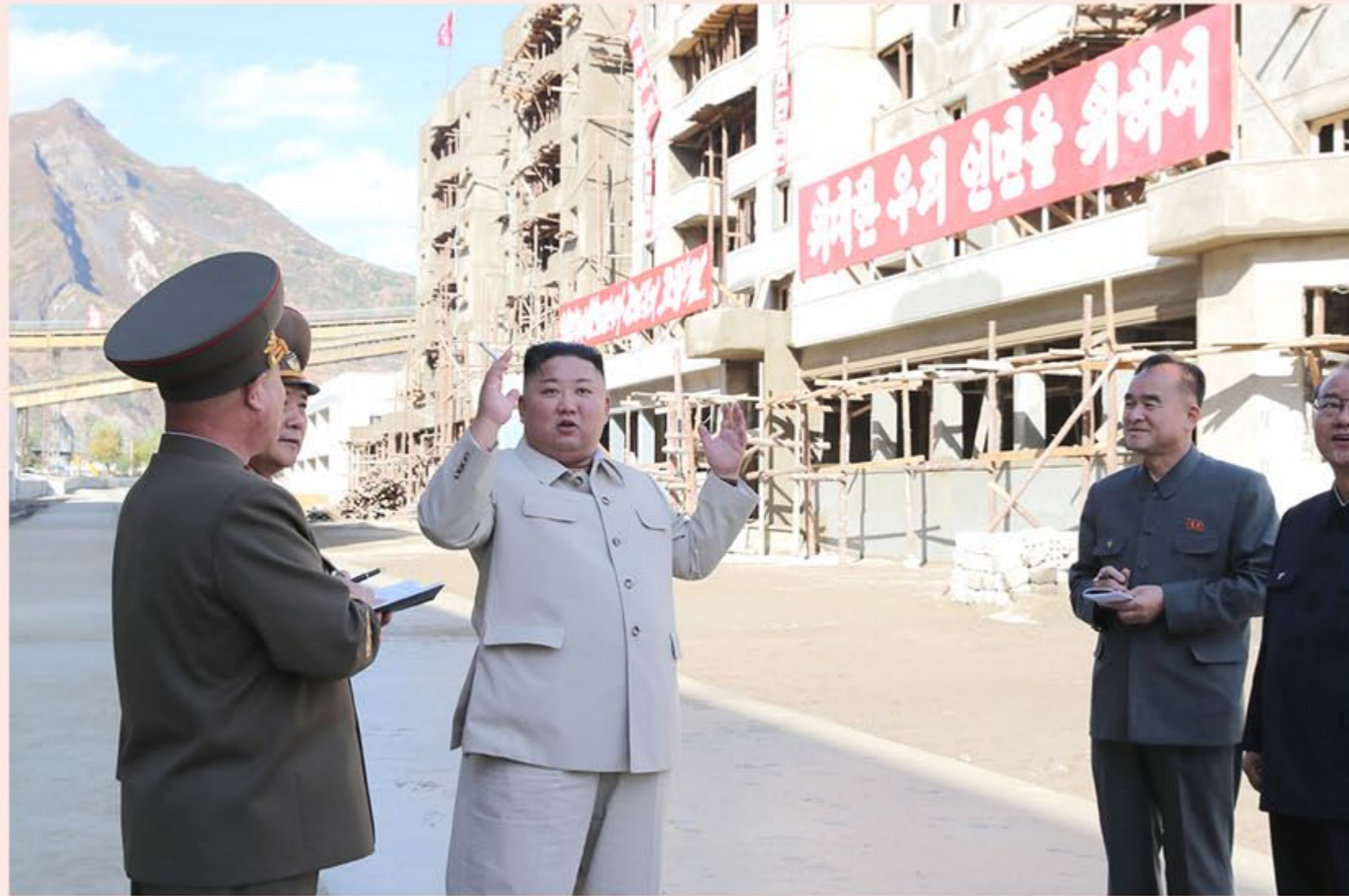
At the reconstruction site in the Komdok area of South Hamgyong Province in October 2020
