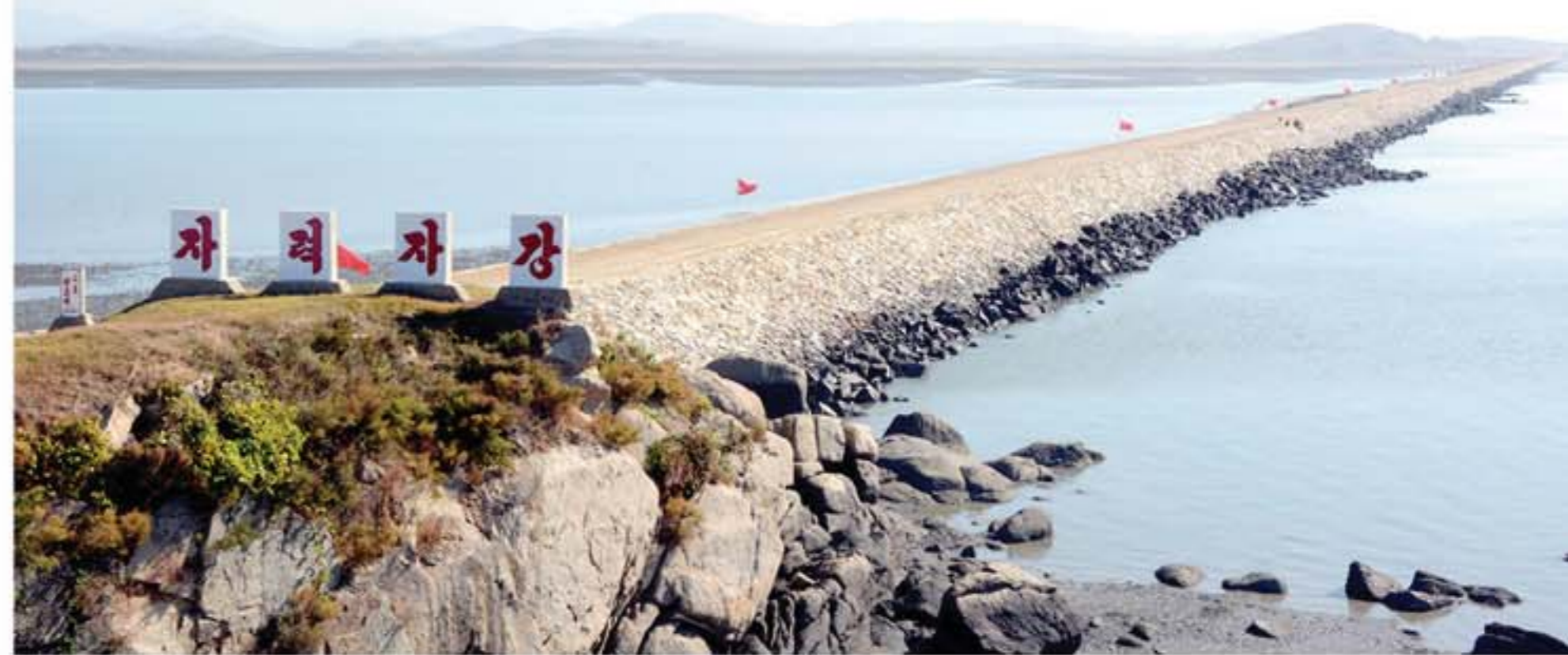
The first-stage construction of the Honggondo Tideland was completed.
